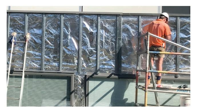
Rear Ventilated Facades have been used extensively throughout the world over many years to provide a natural, energy efficient method for cladding commercial and residential buildings.
